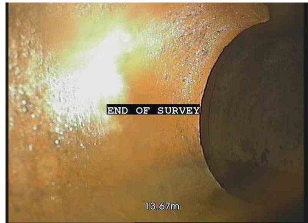
2, 00:01:54, 13.67 m Finish node, manhole, reference: IC4
