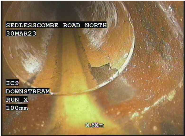
1, 00:00:15, 0.50 m Junction at 6 o'clock, 150mm dia, Interceptor
