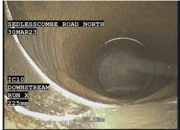
2, 00:01:56, 21.12 m Junction at 6 o'clock, 225mm dia, Backdrop
