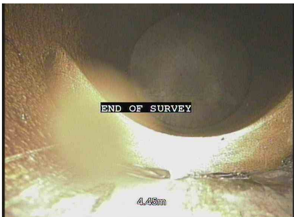
3, 00:00:56, 4.45 m Finish node, manhole, reference: IC5
