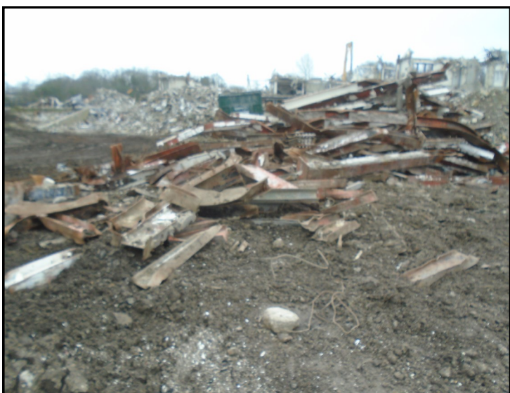
LOCATION OF IC7 OBSTRUCTED UNABLE TO LIFT
