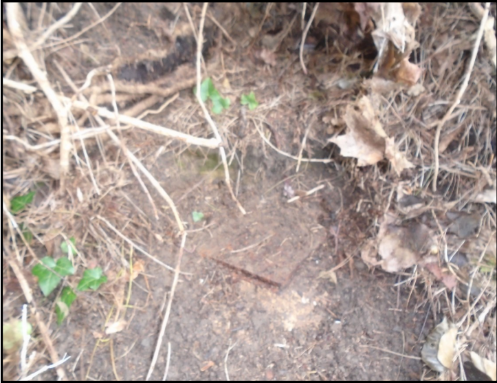
IC11 UNABLE TO LIFT OBSTRUCTED WITH FALLEN TREE
