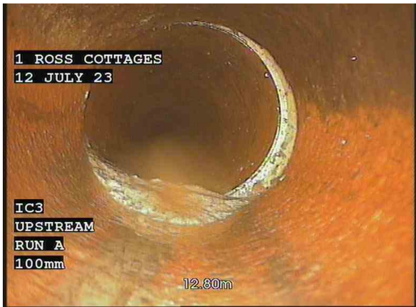
1, 00:01:06, 12.80 m Settled deposits, hard or compacted at joint, 10% cross-sectional area loss, Scale
