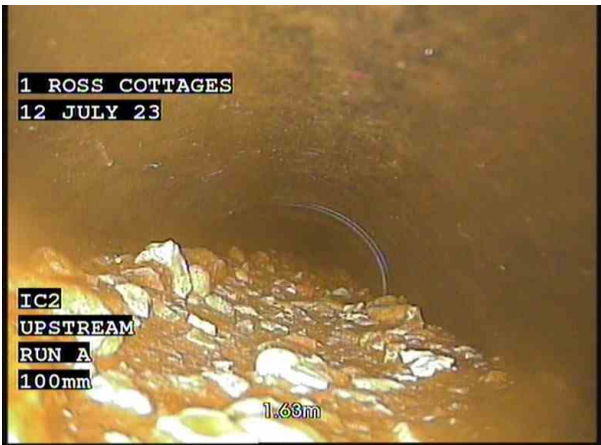
3, 00:00:52, 1.63 m Survey abandoned, Unable to continue
