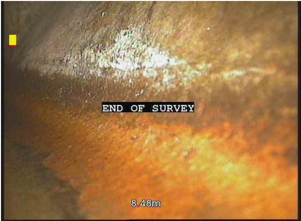
1, 00:00:30, 8.48 m Finish node, manhole, reference: IC3, U.T.L
